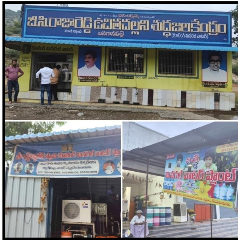
Fig.5.1. Various water filter plants (govt/private) in district
